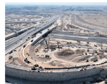
Al Khor Expressway (Qatar)
