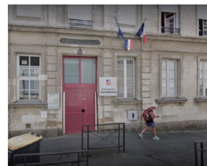
Nursery School Parcheminerie (France)
