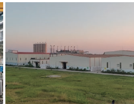
Akij Plastics Chhatak Plant (Bangladesh)
